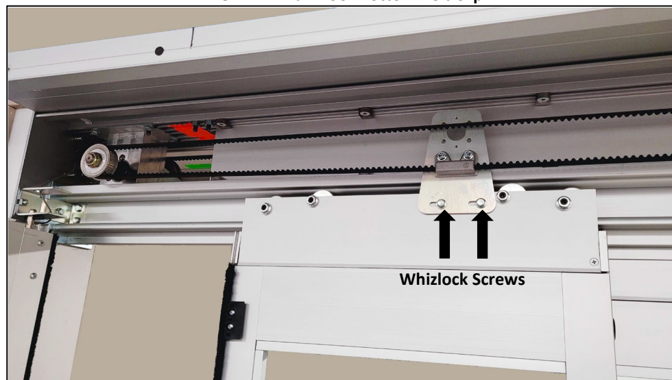
Figure 38 Install the Trail Door Carrier onto the Track
