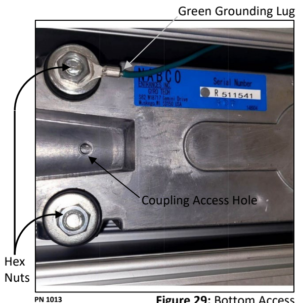
Figure 29: Bottom Access Hole
