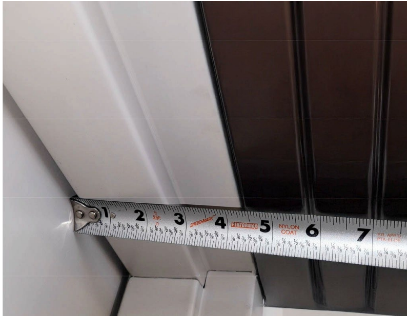
Figure 23: Measure Reveal
